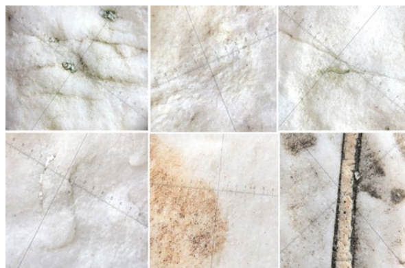
Figure 9: Typical macro defects of the dolomite marble of Madam Song’s Statue in Shanghai. Source: Dai Shibing.
