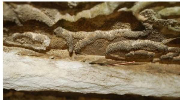
Figure 6: Typical deterioration of dolomitic marble through industrial \text{Na}_2\text{SO}_4 dusts. Source: Dai Shibing.
