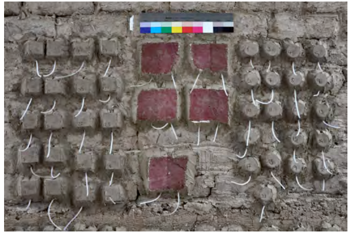
Figure 5. Mock-up wall tests. Different grout formulations were injected behind plaster tiles; after several month of curing adhesion and distribution in the void will be analysed/ recorded. (Photo: Gesa Schwantes)
