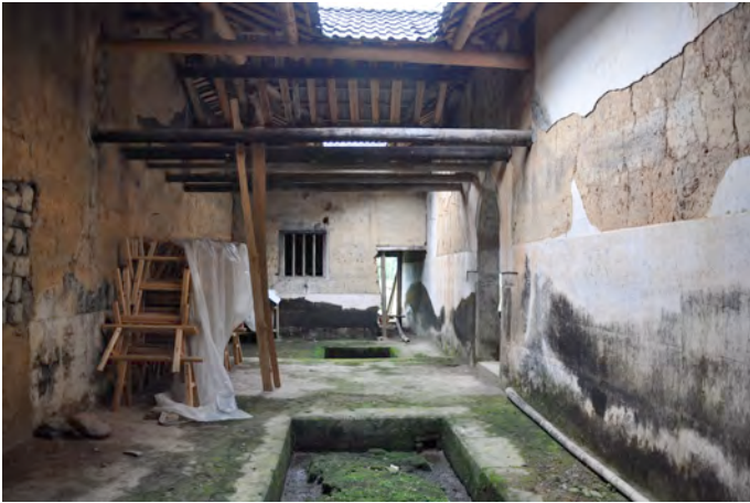
Figure 7. Room on the west side of Liu's Family Ancestral Hall, with clay plaster fragments. (Photo: Gesa Schwantes)
