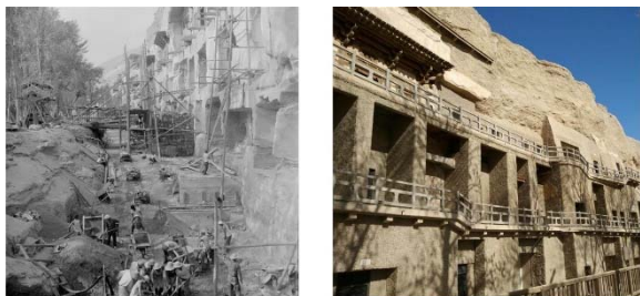
Figure 3: (Left) In 1964, the reinforcement project of external rock wall in Mogao Grottoes was underway. (Right) After the repair, the reinforcement effect of the retaining wall is still effective today. Source: Dunhuang Research Institute.
