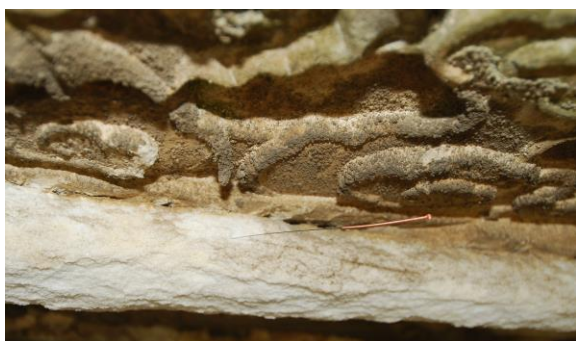
Fig. 6 typical deterioration of dolomitic marble through industrialization (hier \text{Na}_2\text{SO}_4 dusts attacked dolomitic marble), , Source: Dai Shibing
