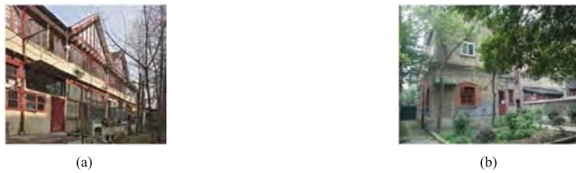
Fig. 1. (a) The south elevation (covered with flat plaster), (b) the north elevation (original render is kept partly)
