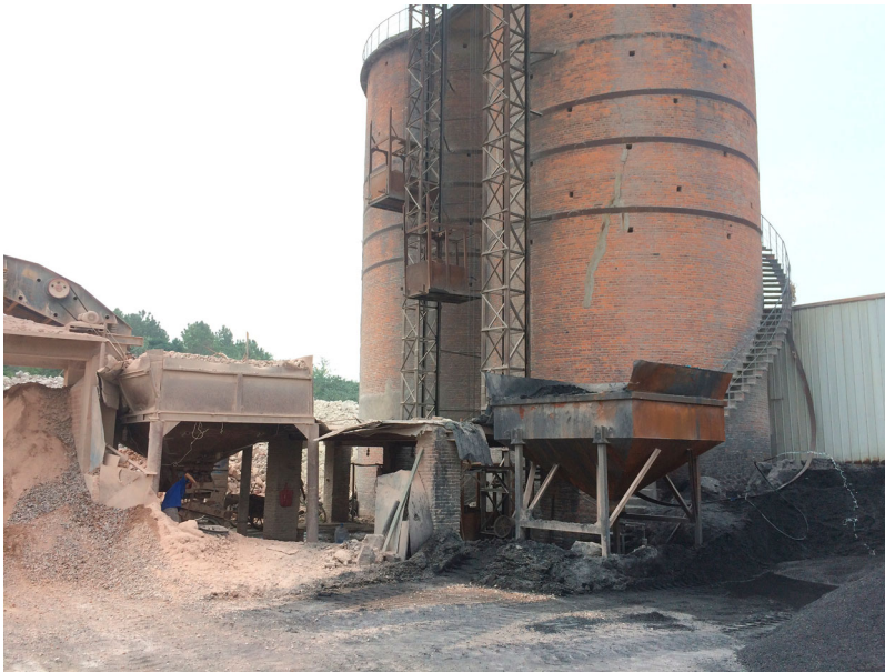
Figure 6. Shaft kiln for lime production, where the quick lime was collected for testing, coal as fuel as described in the Heavenly Creations in the seventeenth century (photo taken in 2016 before environmental upgrading).
