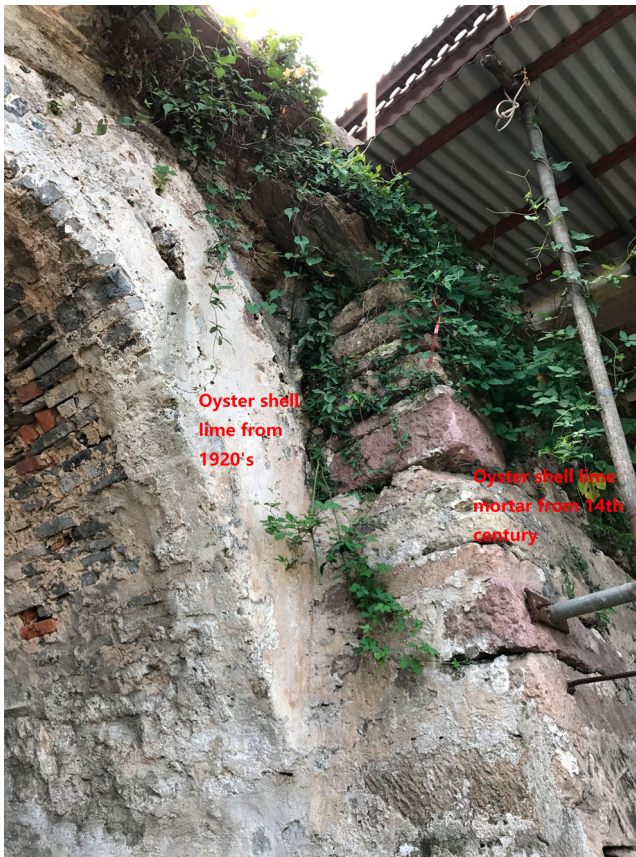
Figure 4. Physical documentation of oyster shell lime for masonry and plastering in East Gate Ruin of former city wall of Taizhou, Zhejiang province, built in 1387.
