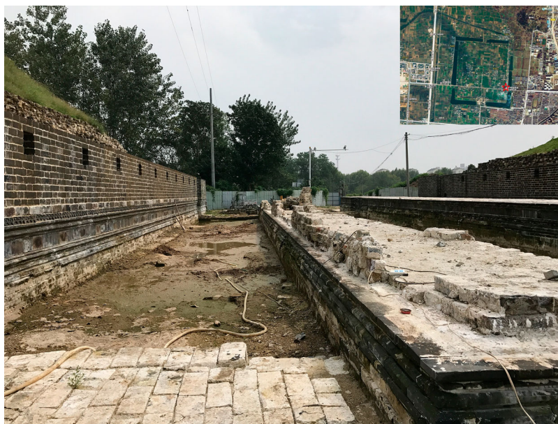
Figure 1. Massive masonry lime in Dong Hua Men Ruins (left) of Central Emperor Palace in Fengyang, Anhui Province, built between 1369 and 1375, at the beginning of the Ming Dynasty.
