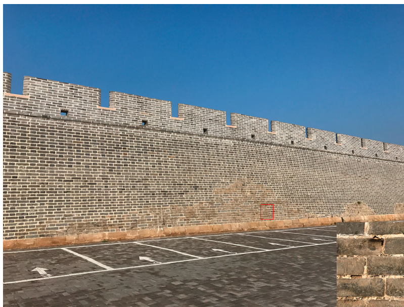
Figure 3. Historic mortar remains in the Great wall of Lao Long Tou in Shanhaiguang City, Eastern Beginning of Great Wall built around 1381, Ming Dynasty.
