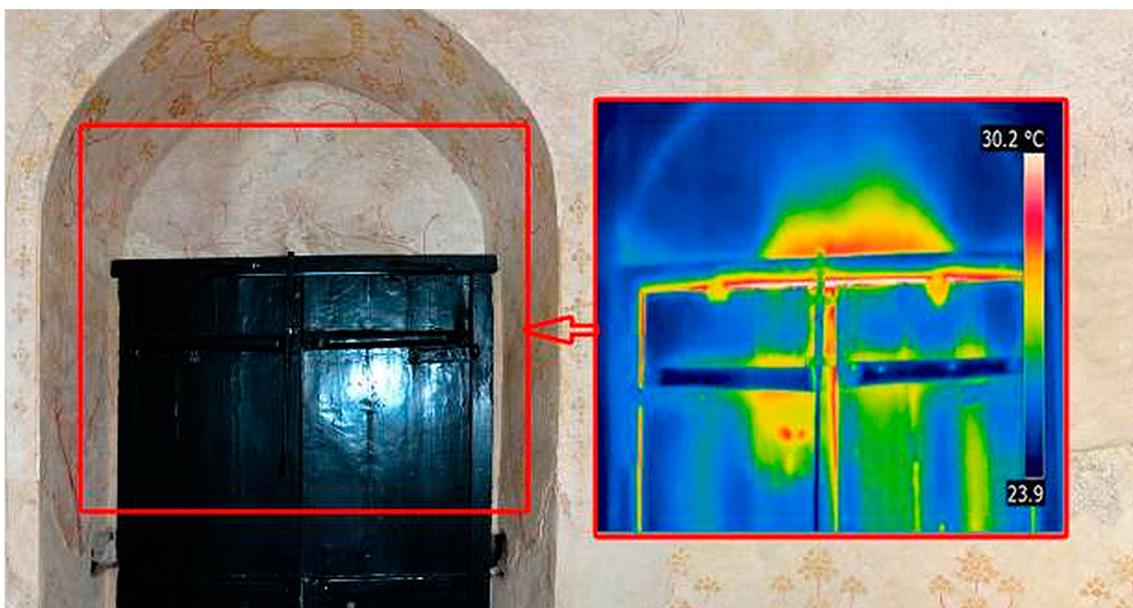
Figure 8 Surface temperature difference of wall paintings shown on thermogram.
