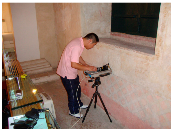
Figure 11 Penetration resistance testing the interior and surface of the wall of the Chapel.
