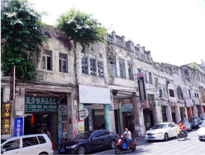
Bild 5: Shop-houses in Haikou, on North Boai Road, before conservation.
