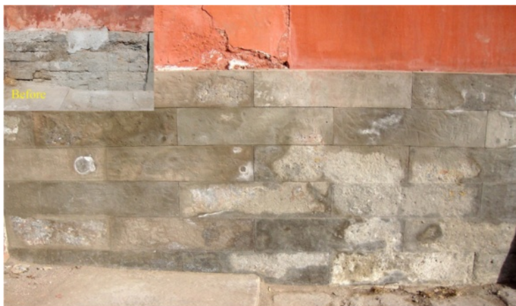
Figure 10 Trail to use lime to restore traditional Chinese green bricks (right after restoration).
