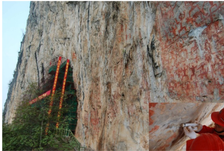
Figure 1 Conservation of Huashan Pictographs during 2009–2013 using natural hydraulic limes as raw material, Guangxi Autonomy.
