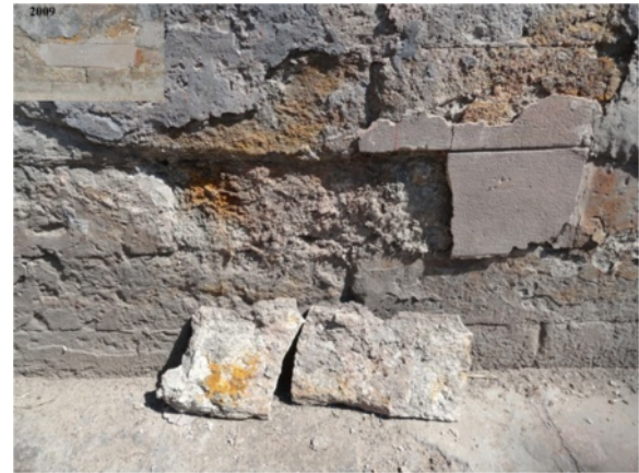
Figure 9 Cement-based mortar applied in 2002 to restore green bricks in Beijing, delaminated in 2012.
