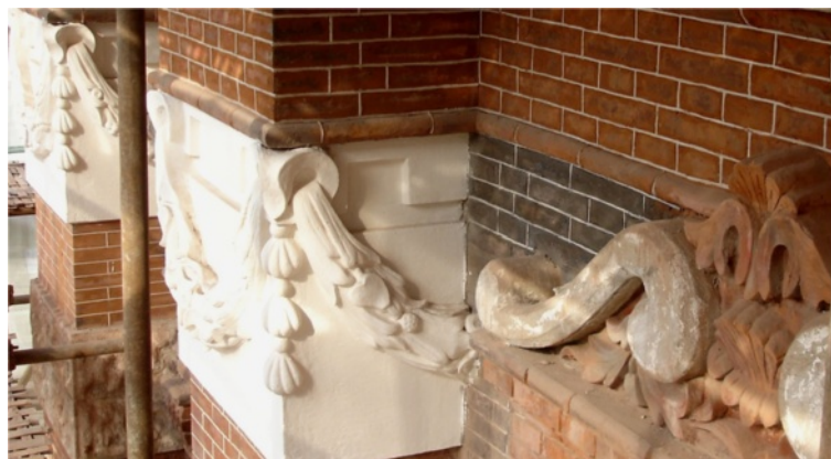
Figure 8 Strawed dispersed lime to restore marble imitated ornaments in Xuhui High School Shanghai (built in 1850).
