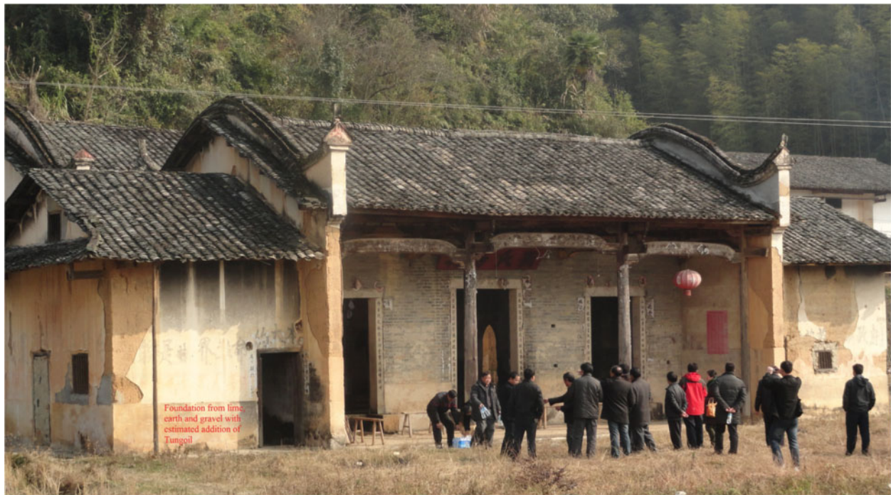
Figure 5 Traditional earthen-timber architecture built in 1824 with foundation from lime, earth and gravel with estimated addition of Tungoil in Jiangxi Province.
