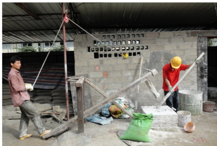
Figure 4 Preparation of lime plaster finishing by tempering for façade restoration in Haikou 2011.
