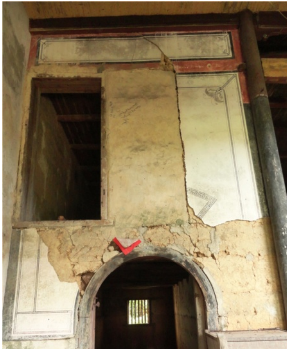
Figure 7 Mural painting of vernacular architecture (early 19 th century) on lime-earthen substrate in Jiangxi Province.
